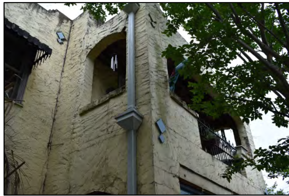
Figure 11. Applied paired diamonds, painted blue, at front elevation
