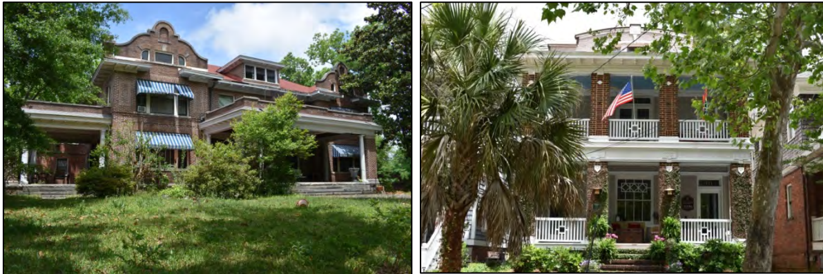
Figure 23: Joseph Hatch Hinton House (1912-1913), at left, and duplex of Edward E. David, (1911), at right
