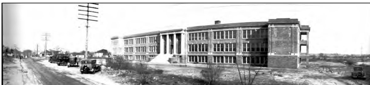
Figure 47: Williston High School under construction, 1931 (photographer: Louis T. Moore; source: http://cdm16072.contentdm.oclc.org/cdm/singleitem/collection/p15169coll6/id/136/rec/20 )
