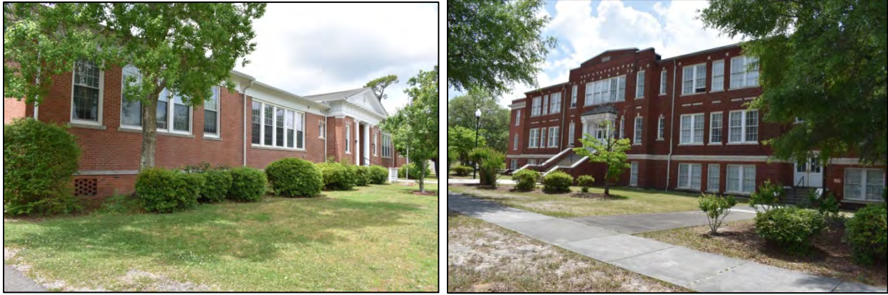
Figure 50: Delgado School, now a transitional living center, at left; William Hooper School, now the Hooper School Apartments, at right
