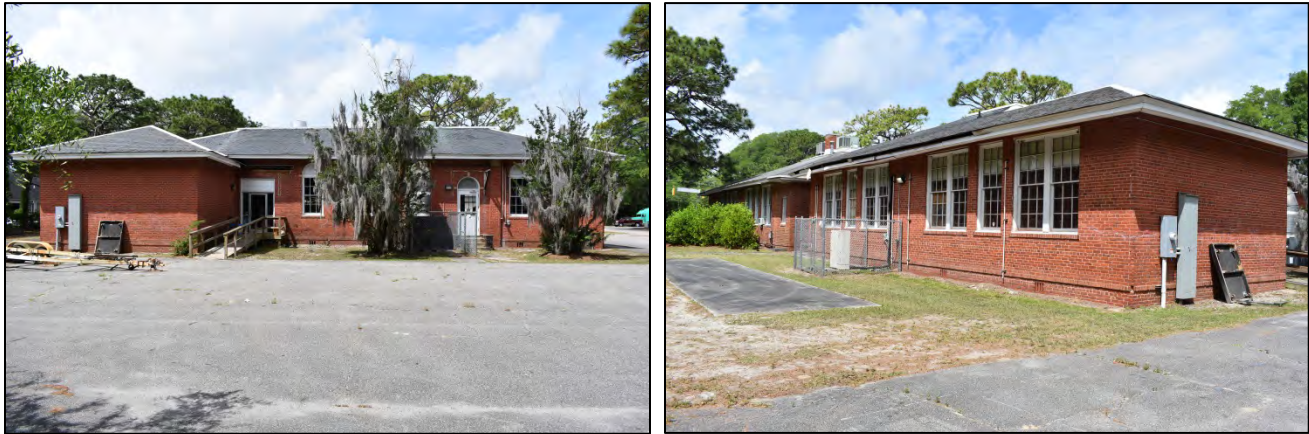
Figure 35: At left, rear elevation with long auditorium and blank walls of rearmost classroom and, at right, south elevation with added classrooms at center and right and original block at far left
