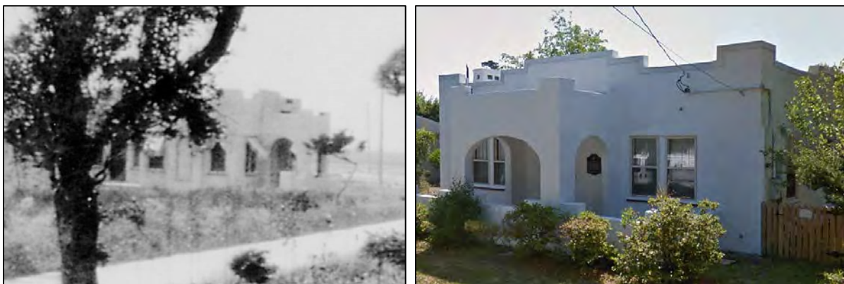
Figure 24: Shore Acres House (1928) in Wrightsville Beach just after construction in Louis T. Moore photograph, at left, and in June 2016, at right
