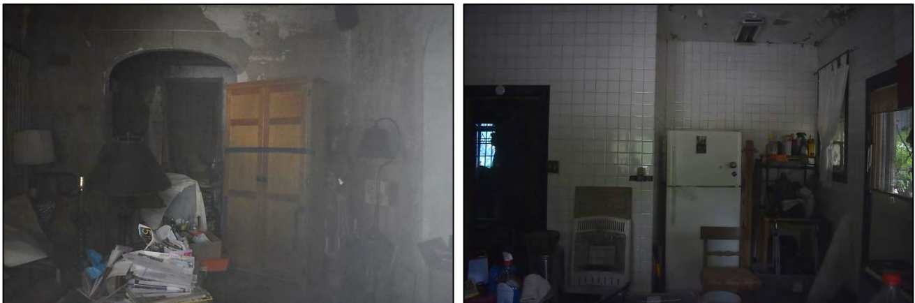
Figure 12: First-story—southeast front room, at left, and northeast front kitchen, at right
