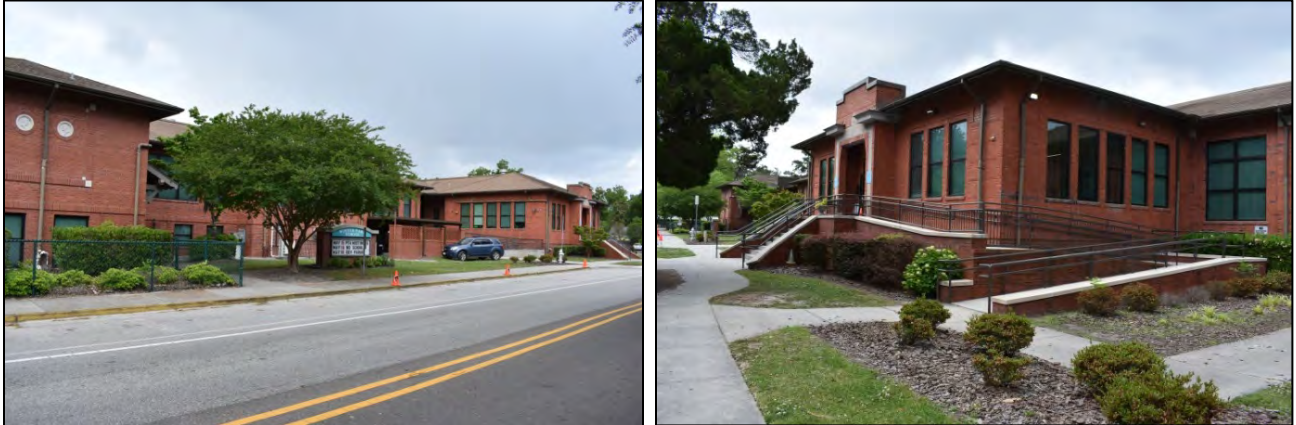
Figure 51: Winter Park School, 1912 and later; original central block easily discernable in both images
